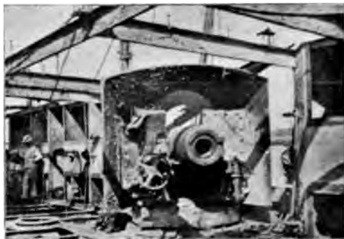
The MARIA TERESA. Showing hole in 5.5-inch gun-shield, inner view.
